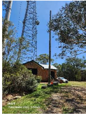
Beacon Pole Overall View
